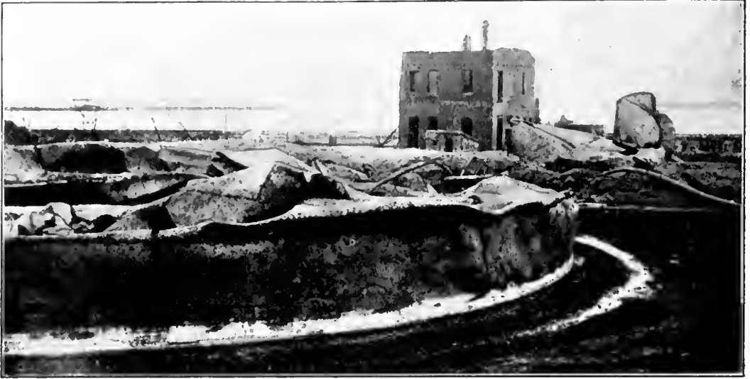
OIL TANKS DESTROYED AT TSING-TAU,
